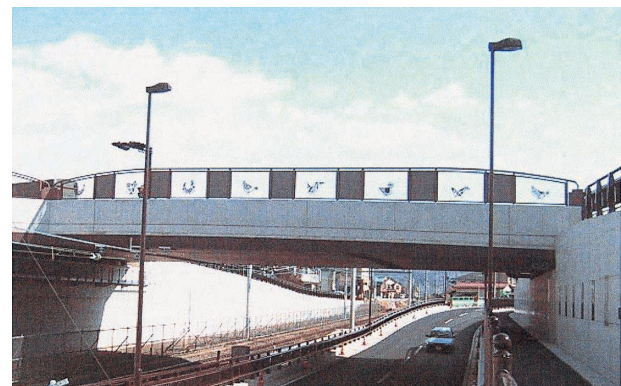
Photo 6 Appearance of Maruyama-bashi Bridge applied with e-RUS treatment and pre-coat system (Okaya City)
