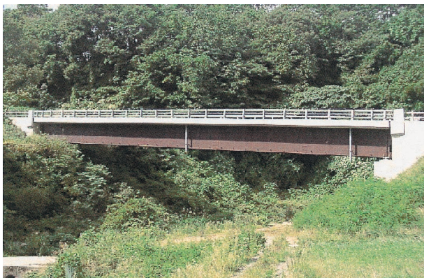
Photo 2 Appearance of Shinkouji-oohashi Bridge made of Ni added weathering steel (JFE-ACL Type2)
